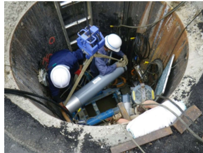
Shaft for Separable launching and installation of thrust jack
