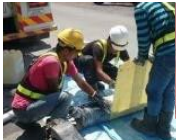
Resin Patch Repair
