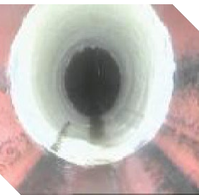
Resin Patch Repair
