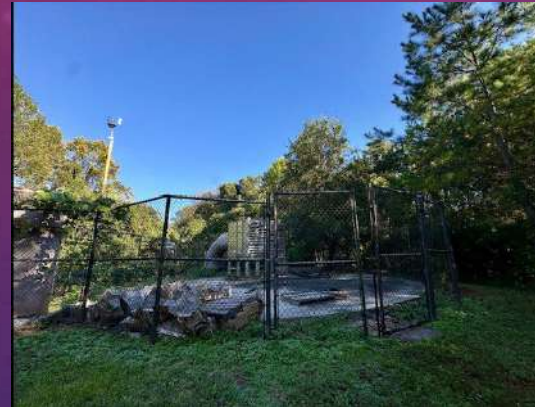
Johnson Ferry Rd. Access Shaft with Odor Control Equipment
